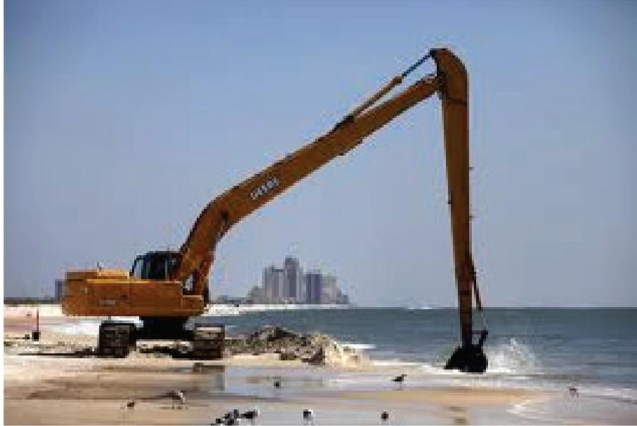
**Figure 5.17** Track hoes Used for Excavation of Tar Mats at Tidal Interface
